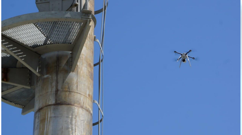
Drone Used by AETOS Group for Flare Stacks Inspection [3]
