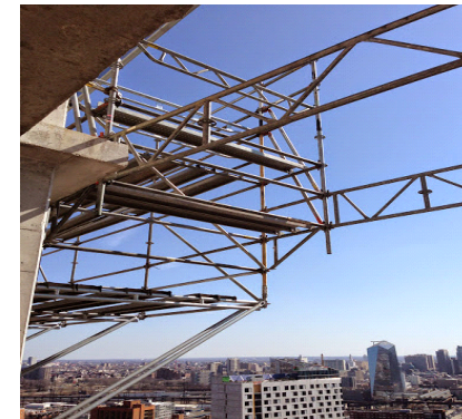
Cantilevered temporary work platforms
