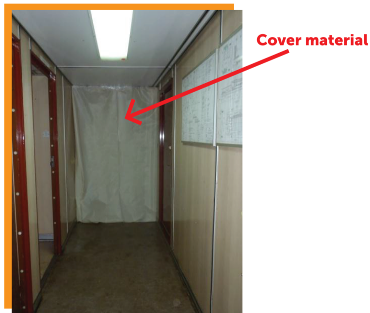
Figure 6.3: Isolation of asbestos removal area
