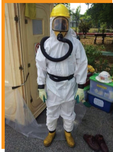
Figure 6.9: Asbestos removal worker wearing a full PPE and respirator
